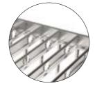
No need for blocking between joists at ends. The boundary joist takes care of that.
